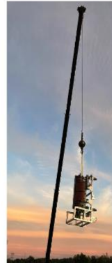
Vertical Lift: "Single Point Lift"
